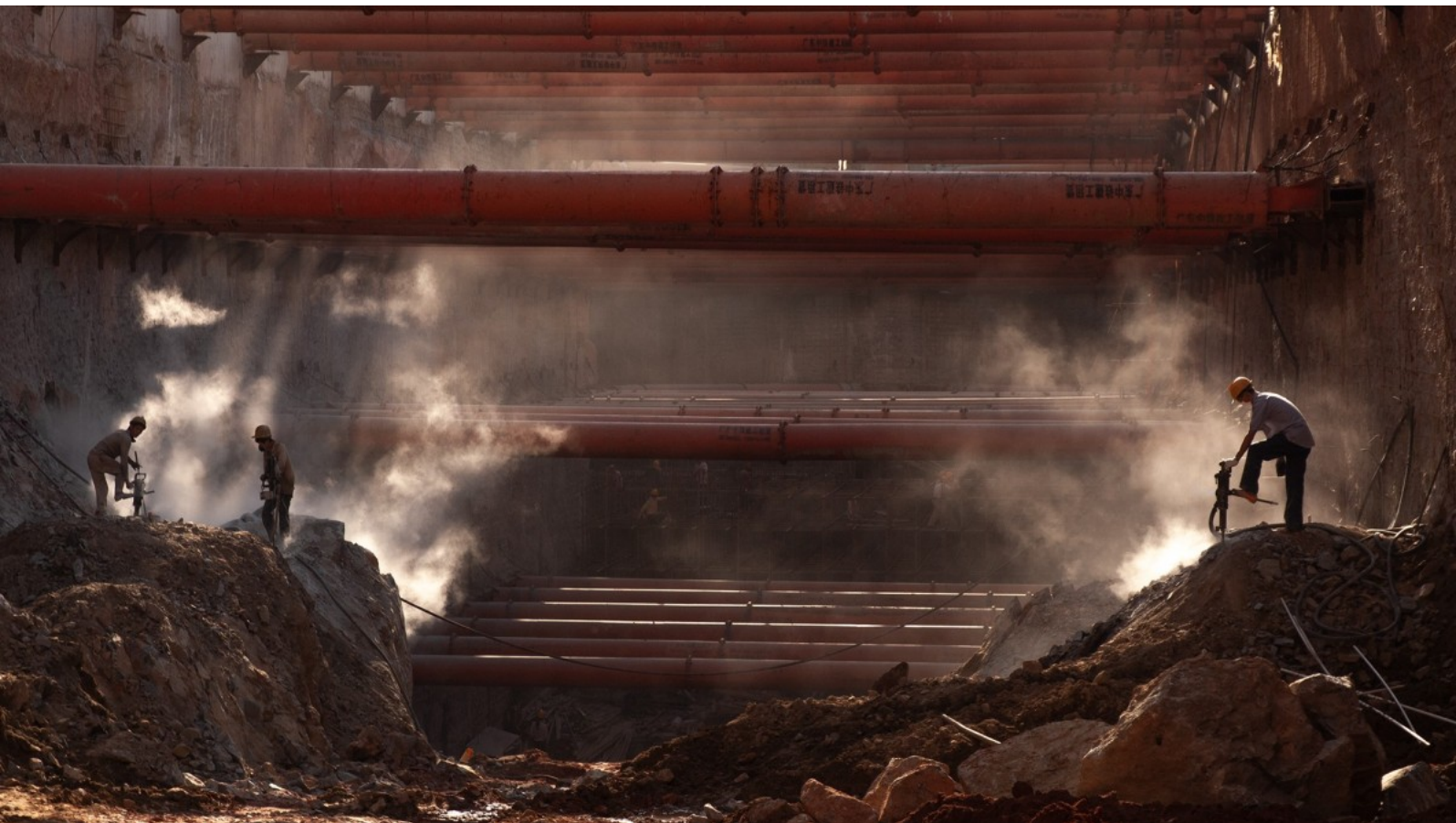
Salon 5 - PSA GOLD MEDAL - CONSTRUCTION WORKER by ZHITANG ZHONG (CHINA)
